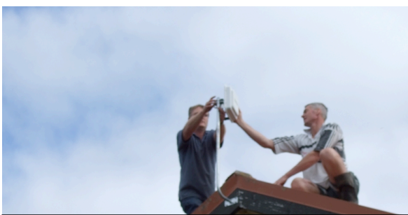
Wayne and Rex During Installation
